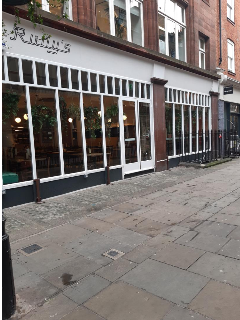
View of the ground floor elevation along Meard Street
